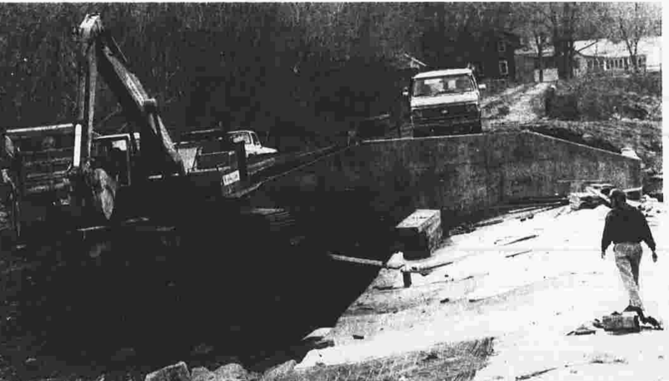
Bolton dam on schedule Left, Joseph Wilson, an employee of G.L.C. Construction Co., caulk seals in the spillway at Lower Bolton Lake Dam. Workers say the dam reconstruction, which is being overseen by state Department of Environmental Protection, is on schedule. The project is expected to be finished by the end of the year. Above, a dump truck crosses the earthen dam, headed toward the spillway reconstruction work going on at the southeast end of the lake. Below, a worker observes another moving earth as he walks along the spillway, which has been under reconstruction since early September.
