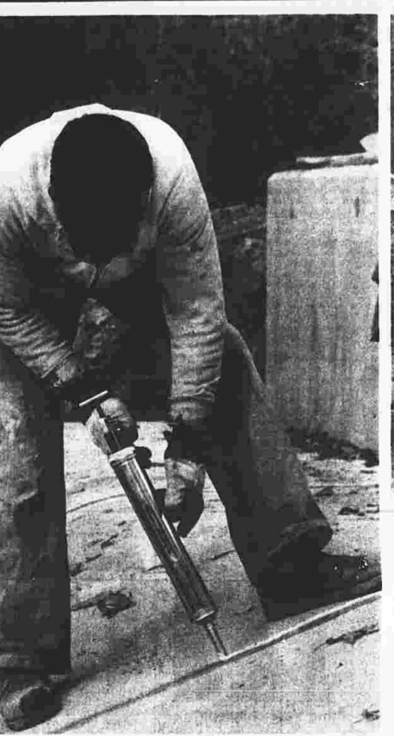
Bolton dam on schedule Left, Joseph Wilson, an employee of G.L.C. Construction Co., caulk seals in the spillway at Lower Bolton Lake Dam. Workers say the dam reconstruction, which is being overseen by state Department of Environmental Protection, is on schedule. The project is expected to be finished by the end of the year. Above, a dump truck crosses the earthen dam, headed toward the spillway reconstruction work going on at the southeast end of the lake. Below, a worker observes another moving earth as he walks along the spillway, which has been under reconstruction since early September.
